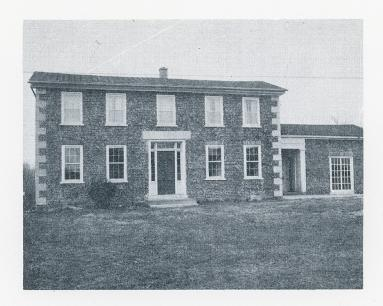
The cobbles are lake-washed stones and colors have been sorted out. In the front wall black stones are used, red stones in the south wall, while white and gray stones are used in the north wall of the main portion of the house. These colors are mixed with prevailing tan stones to give a continuity.
